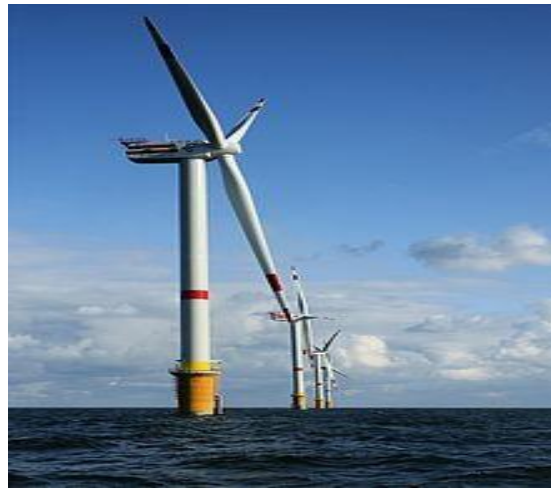
Fig: 3.2 Offshore wind farm using 5mw turbines repower m5 in the north sea off Belgium
