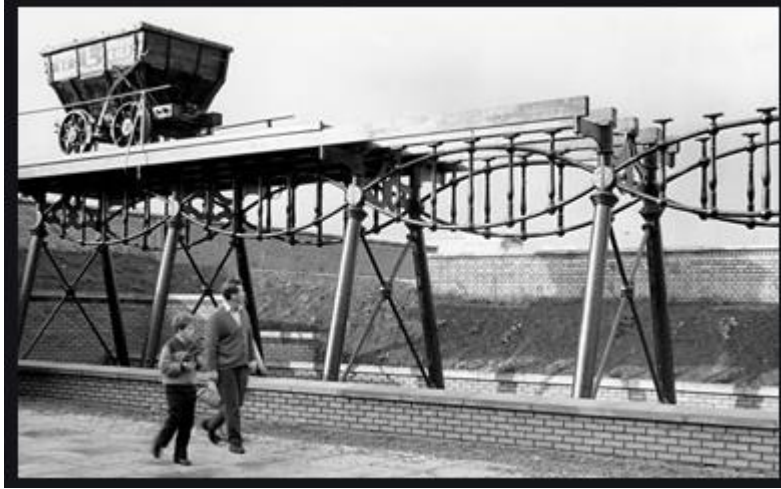
Fig 1.6 lenticular truss
