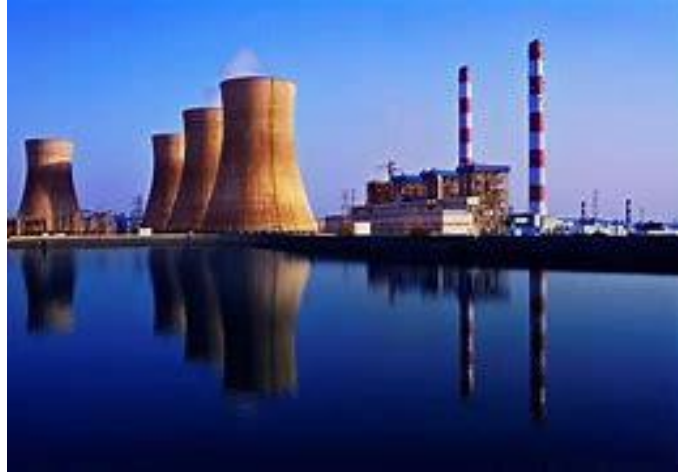
fig 1.4 thermal storage plant
