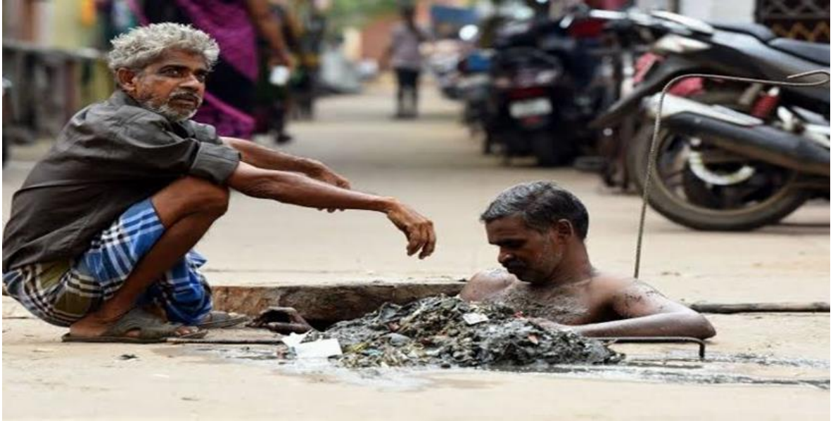
Fig 1.2 Manual drain cleaning
