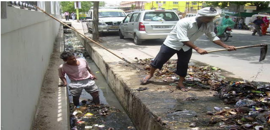
Fig1.1 Manual gutter cleaning to remove solid waste
